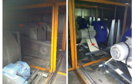
Figure H-1 - EC Plug Fan Upgrade
